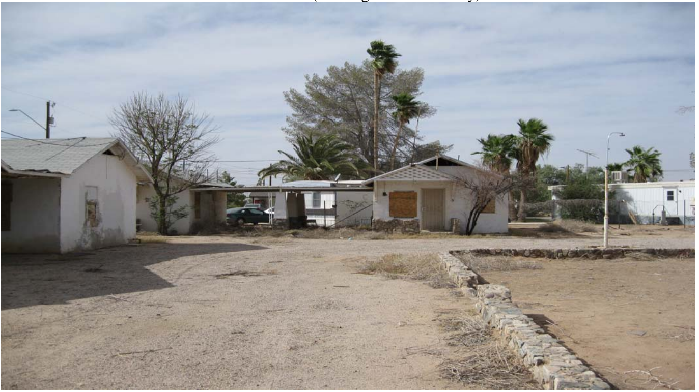
Courtyard with the 8 cabins (all vacant and in poor condition).
